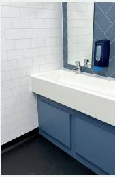
"We used the Vepps IPS system here as we had a tight timeline to get 3 floors / 6 areas done in the summer holidays, so the pre-plumbed system reduces installation times." Additionally, the system offers safe and secure duct spaces, with easy access for ongoing maintenance, ensuring a reliable and practical solution for the school.
